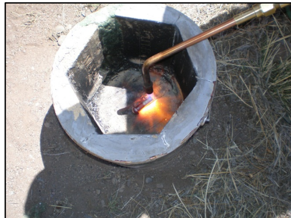
Rivet being heated prior to installation.
