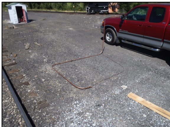
Gene and Bill Bailey working on making the ground loops for the north and south side of the hoist house.
