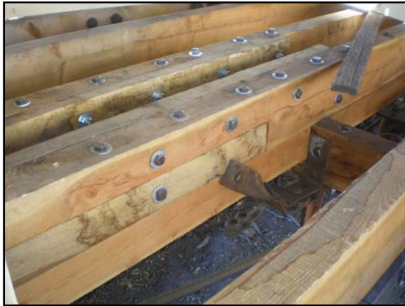
Sills spliced and bolted together.
