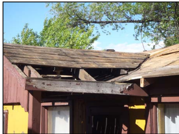
Exposed roof showing rotted wood that needed to be removed and replaced.
