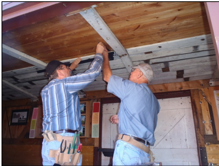
Wayne Huddleston and Bob Hawkins installing a piece of track for the track lighting.
