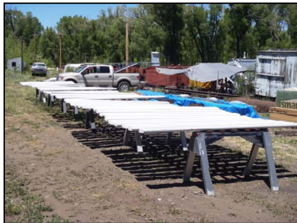
Painted 2 x 8 ship lap decking drying.
