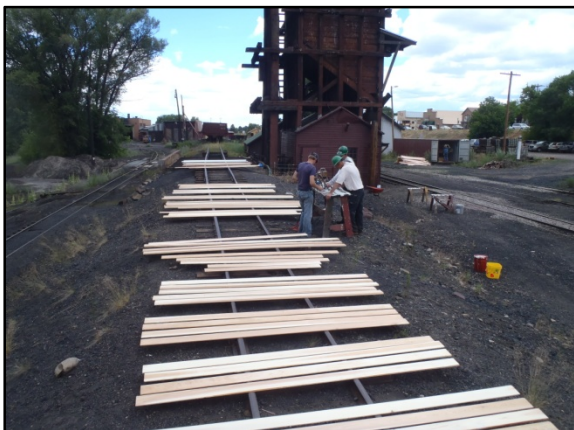
New siding spread out for priming.
