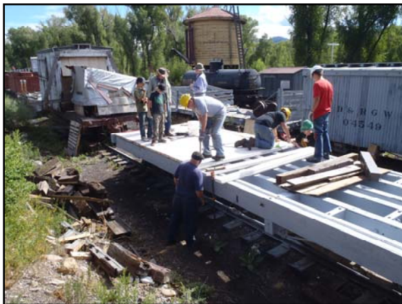
The whole crew including 2 Boy Scouts installing the ship lap deck planks.
