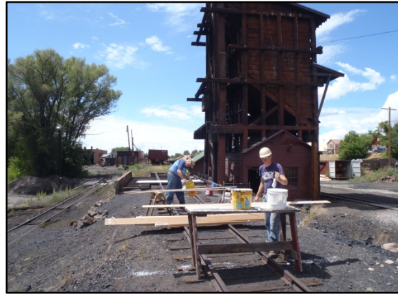
Herb Knoesel and Ron Schmitt priming new siding. They soon changed from hand painting to a spray gun.
