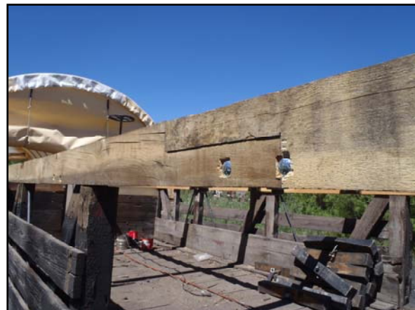
A spliced upper side sill has been installed.
