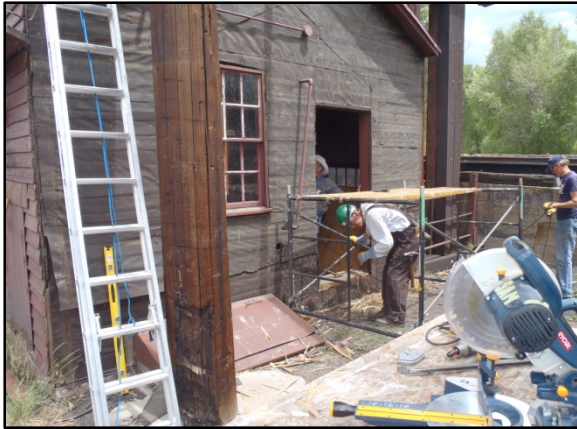
Old siding has been removed from the south side of the hoist house.
