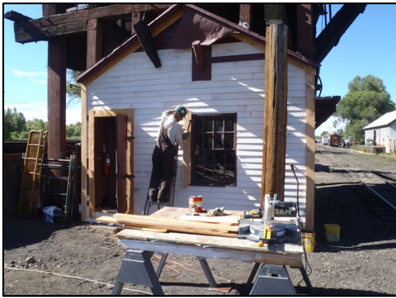
Team Leader John Sutkus nailing the trim around the window of the north side of the hoist house.
