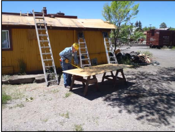
Team Leader Phil McDonald measuring a sheet of 5/8" CDX plywood to be cut to the length.
