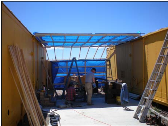
Temporary wind screen under construction. The screen was needed to cut down on the wind for the welders, especially the MIG welder which uses a gas mixture for its flux.
