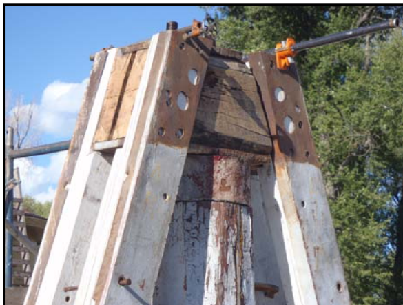
Crown assembly in place ready for holes to be drilled and bolts installed.
