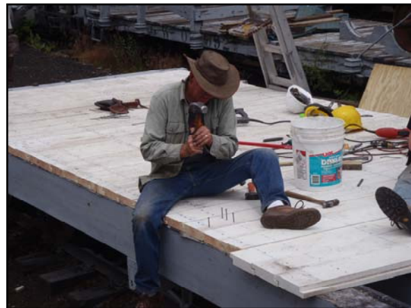
Team Leader Russ Hanscom using a short handled “8 pounder” to nail the 40d ring shank nails into prior drilled pilot holes.
