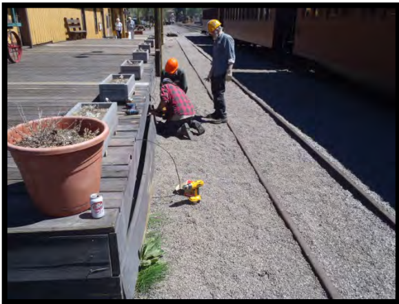
TL Ron Lira, Alan Robson & Herbert Druby removing a 2 X 12 that was nailed on and replaced the nails with screws.
