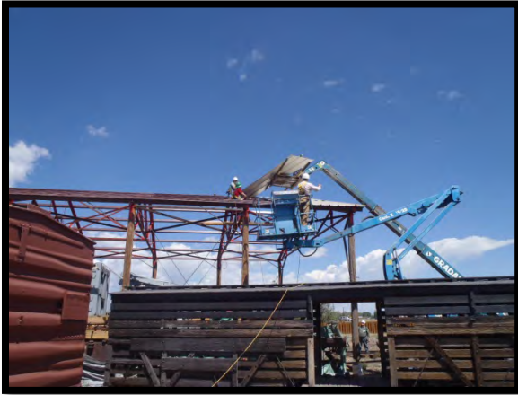
Another sheet being lifted up to the roof.
