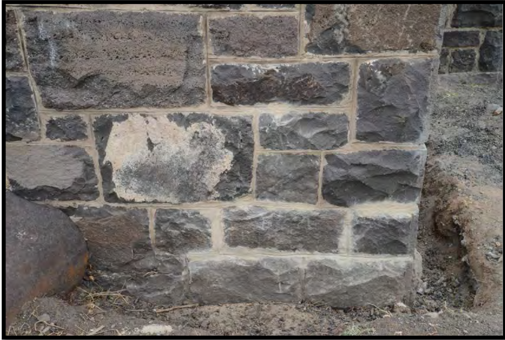
Figure 1: Trench work and repointing at lower NW corner of North wall.
