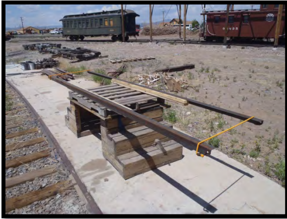
Platform made by Friends members to keep the roof sheathing panels from bending.
