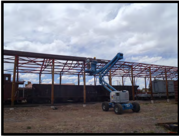
Purlins being installed by two different 2 man crews.
