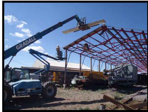
Second roof panel being lifted into place.
