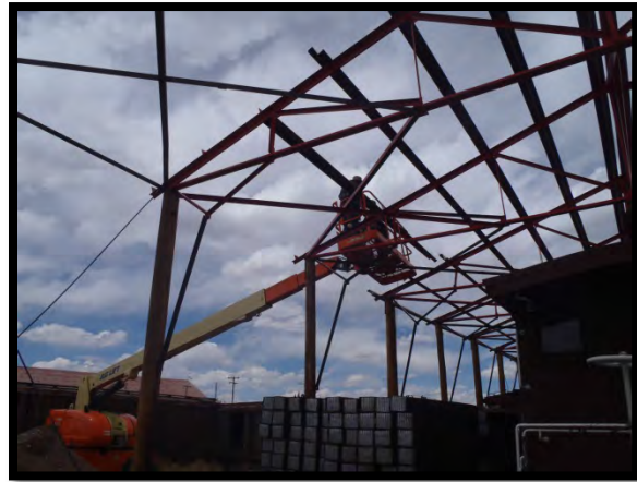
Purlins being installed by two different 2 man crews.
