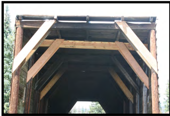
New angle supports installed.
