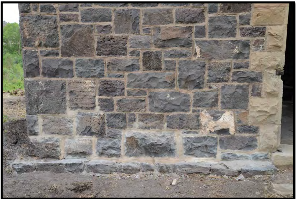
Figure 2: Repointing of lower SE corner of East wall. Foundation stones were exposed by trenching.
