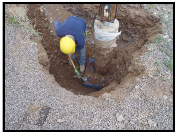
TL Russ Hanscom removing dirt at the base of the column.
