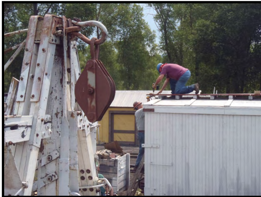
TL Craig McMullen holds a bracket in place as Dan Sandt screws the roof walk board to the bracket.
