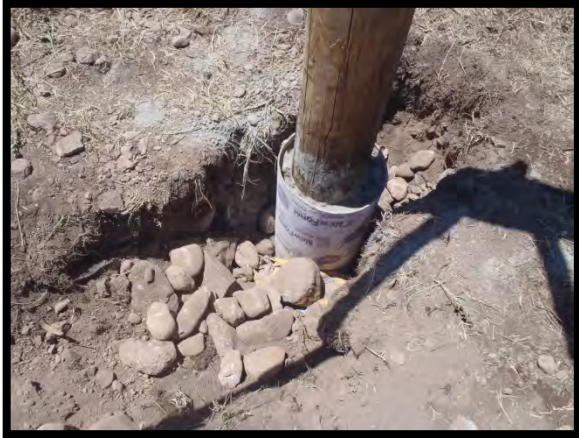
Gate post set and will be backfilled in Session E.
