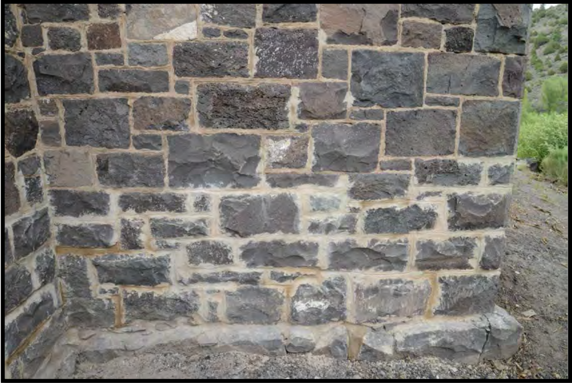
Figure 3: Foundation stones and repointing of lower SW corner of West wall. Dark colored mortar was still wet when photo was taken.
