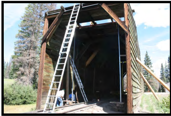
Steel supports being put in place.
