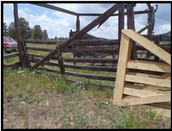
Gate in the process of falling down – old gate will be removed and new gate installed in either Session E or F.
