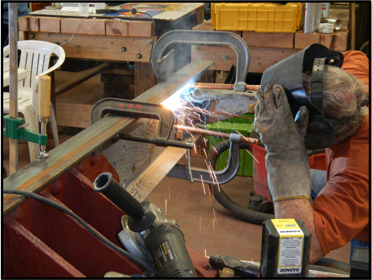
Russ Hanscom welding new steel on DGB #783 end sill.
