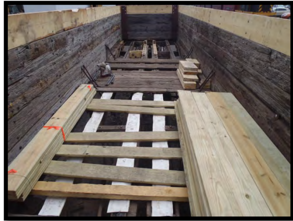
Protective rubberized strips (in white) has been placed over the sills to protect them as much as possible against the elements.
