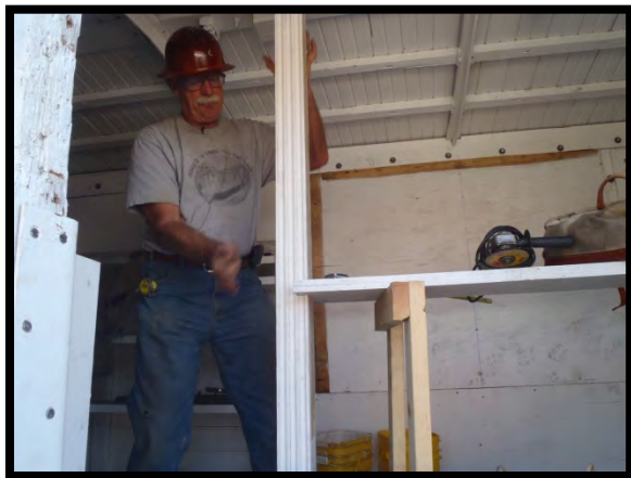
TL Craig McMullen has just finished tapping bolts through the car that holds the overhead door railing as Patricia Sandt tightens up the nuts on the inside of the car.
