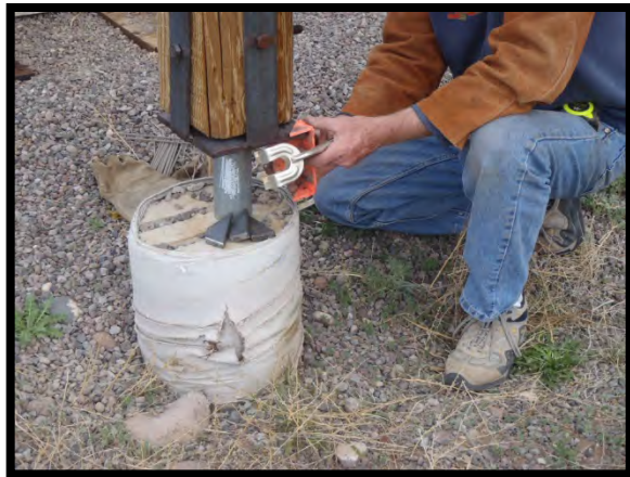
TL Russ Hanscom clamping piece in place to make sure gussets are in correct place and lined up for welding.
