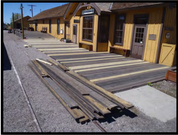
A pile of old 2 X 6's that have been removed and part of the new ones installed.
