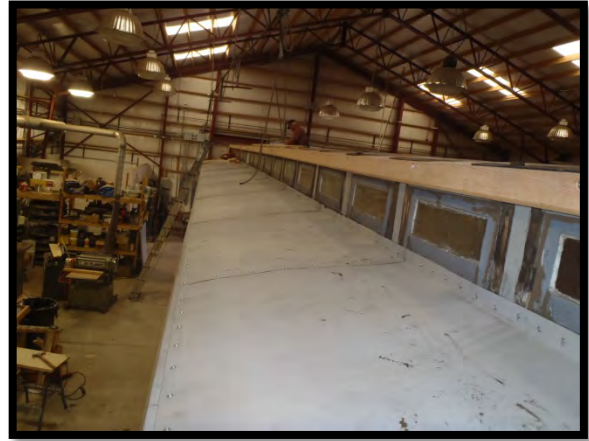
Pre-bent sheet metal roofing with roofing tar and attached with a combination of roofing nails and wafer head self-tapping screws.
