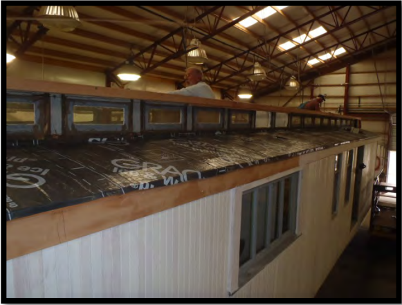
Grace ice and water shield over wood on the side roofs.
