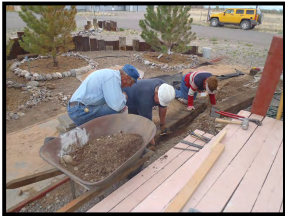
Jim Sublett, John Engs and TL Naomi Sublett work getting tie in place as an edge for the pavers.
