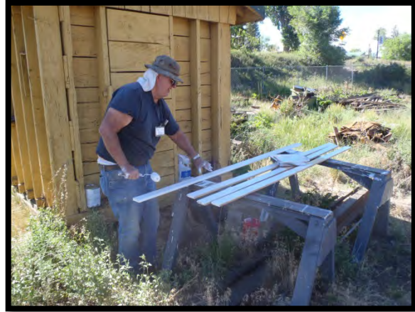
Jon Weiss primes new tongue and groove siding.
