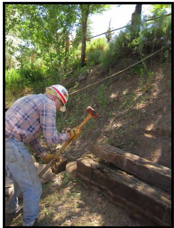
Walt Duncan hammering rebar to stabilize the railroad ties.
