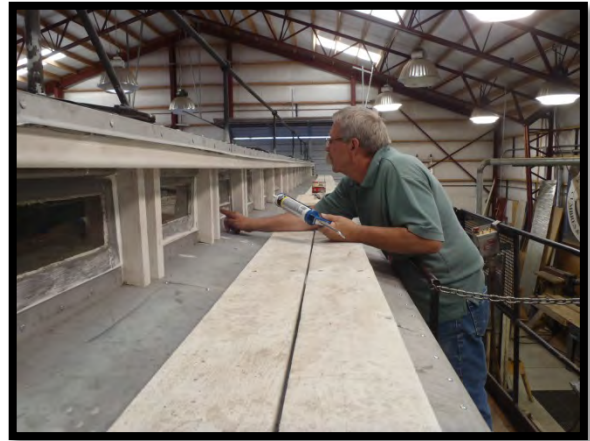
Roof walk was installed and in Session D Mick O'Nele does some caulking on the clerestory windows.
