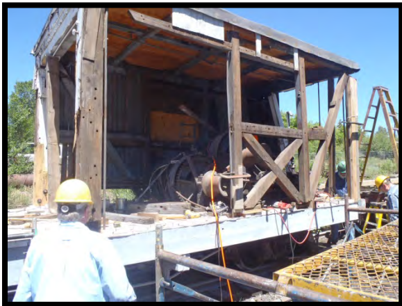
Side of cabin with rotted wood removed.
