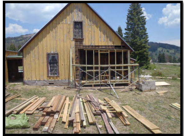
After demo, new framing has been done with full 2 X 4's that were used originally.
