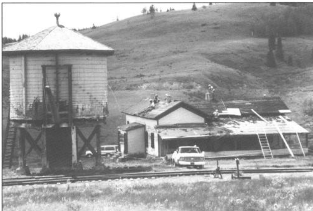
This was the first summer that a Friends crew worked at Osier. Volunteers are removing old shingles from the section house roof in preparation for installing roofing paper as temporary protection over the winter. July 1993. Photograph by Doris Osterwald.
