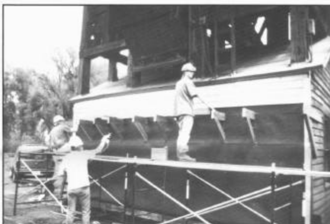
In the Chama yard new siding was placed on the west wall of the coal tippie machinery room. July 1993. Photograph by Jim Gross.
