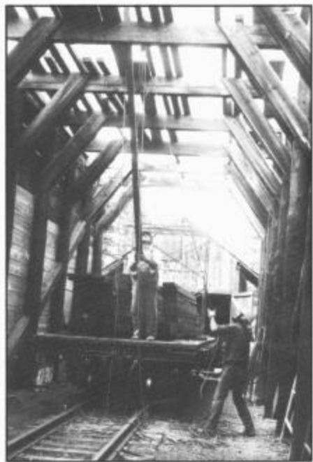
At the Cumbres snowshed, a block and tackle was used to raise decking material from the flat car to the roof. July 1993. Photograph by Terri Shaw.
