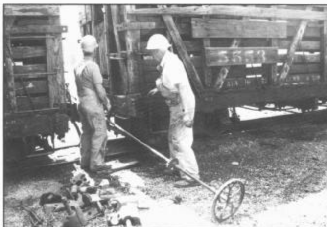
At Chama the brake rigging was reattached to one of the double-deck sheep stock cars donated to the railroad by the Friends . The brake linkage was disconnected years ago when the car bodies were separated from their trucks. July 1993. Photograph by Jessica Ratliff.
