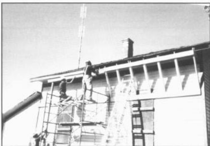
Installing temporary knee braces on the east side of the section house at Cumbres to support the roof and eaves, which were collapsing because of the winter snow load. August 1993. Photograph by Art Nichols.
