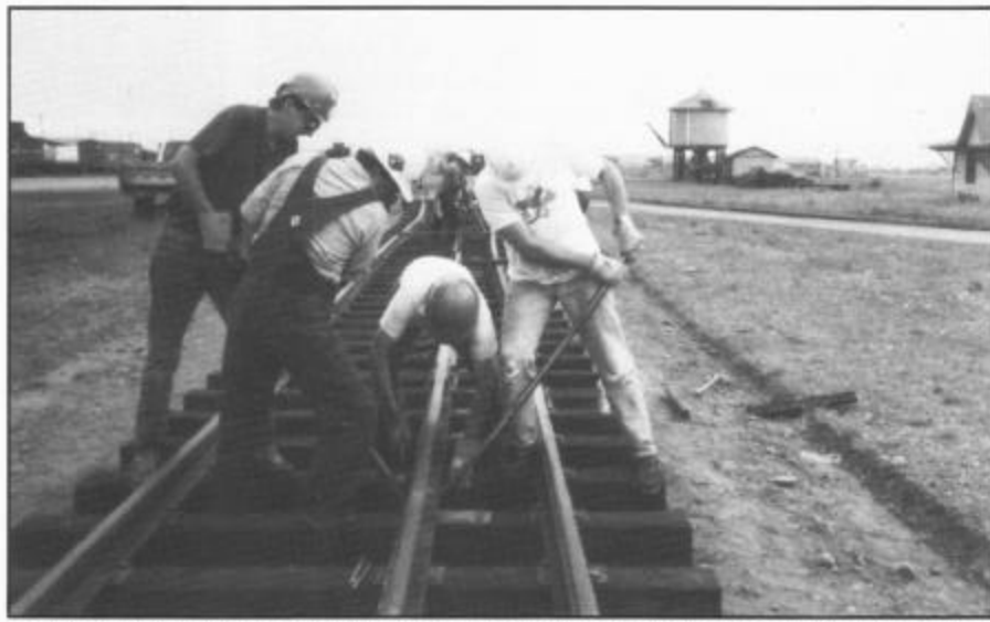
In August 1990 a volunteer crew, assisted by Kyle Railway employees, installed a dual-gauge (4 feet 8½ inches and 3 feet) display track in the Antonito yard. Today, this display track is used for two standard-gauge boxcars and a standard-gauge flat car, or idler car, that joins narrow-gauge and standard-gauge cars in dual-gauge service. The D&RGW used dual-gauge track between Alamosa and Antonito until 1970. Photograph by Art Nichols.
