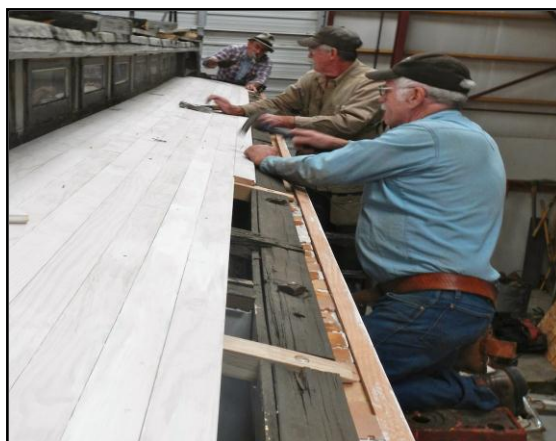
Tim Bristow, Craig McMullen and Chuck Deuker replace roof sheathing
